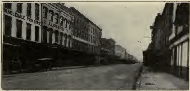
POYDRAS STREET COMPLETED
